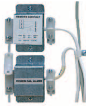
Remote temperature and power failure alarm
